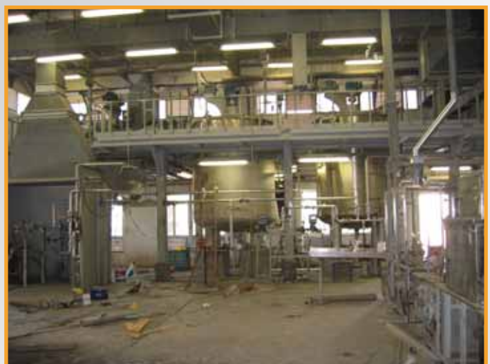
PLANT MACHINERY ERECTION
